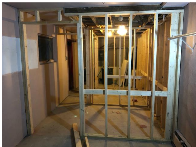
Walls are framed for the new bathrooms
