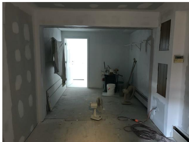
New drywall goes up in the entryway
