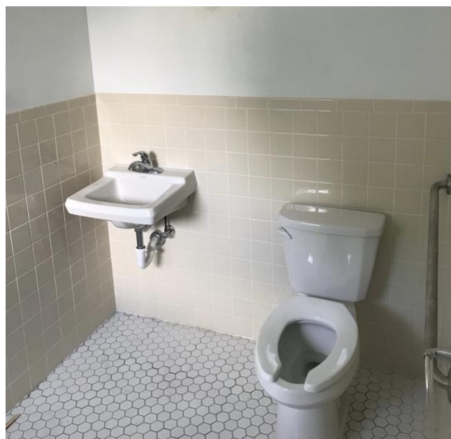
One of the two new bathrooms
